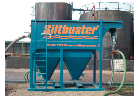
HB50 OWS unit on an industrial creosoting plant
